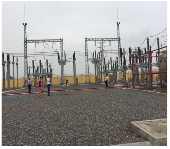
110kV Substation Project – Kim Bang
