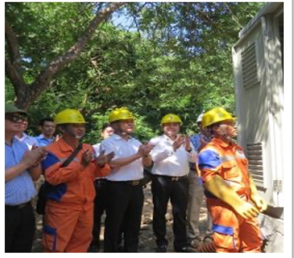
National Grid Power Supply for Reu Island, Cam Pha City, Quang Ninh Province
